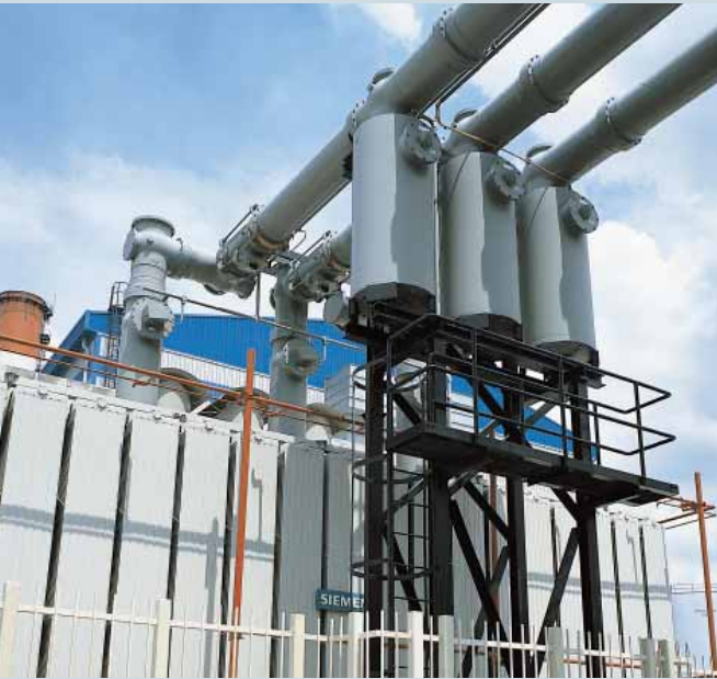
GIS arresters connected to a 420 kV GIS busbar
