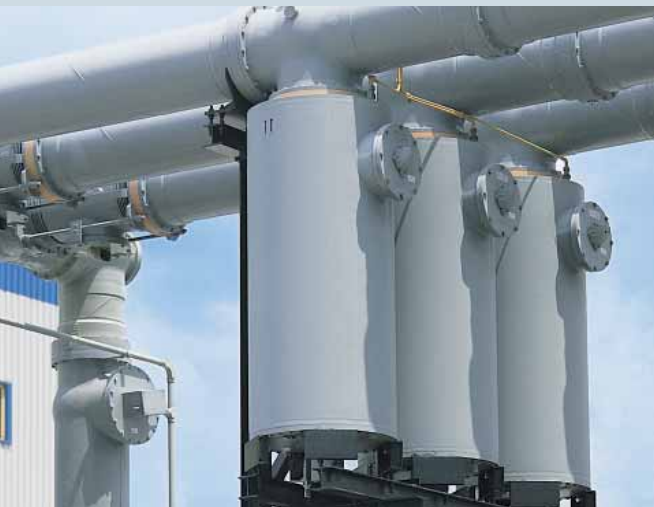
GIS arresters connected to a 420 kV GIS busbar
